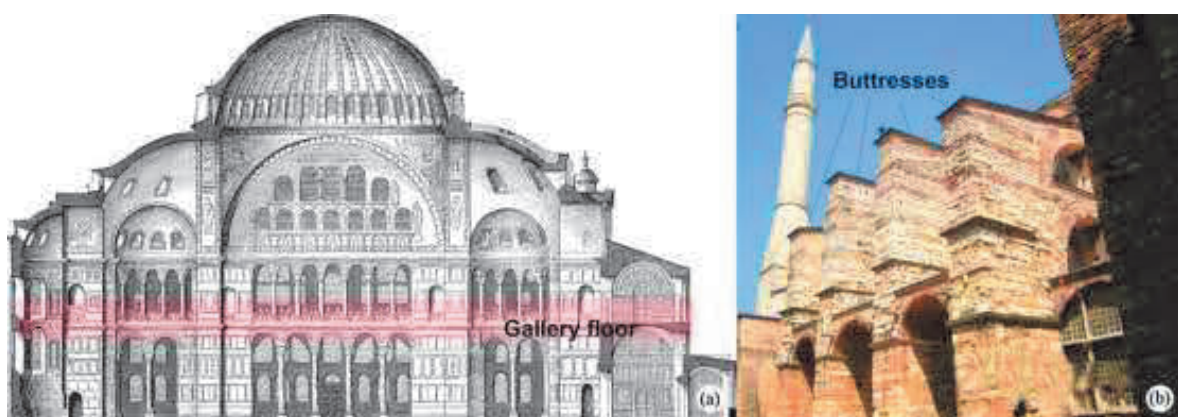
Fig. 1. Hagia Sophia and buttresses added by Architect Sinan (Yalçiner et al., 2017)
