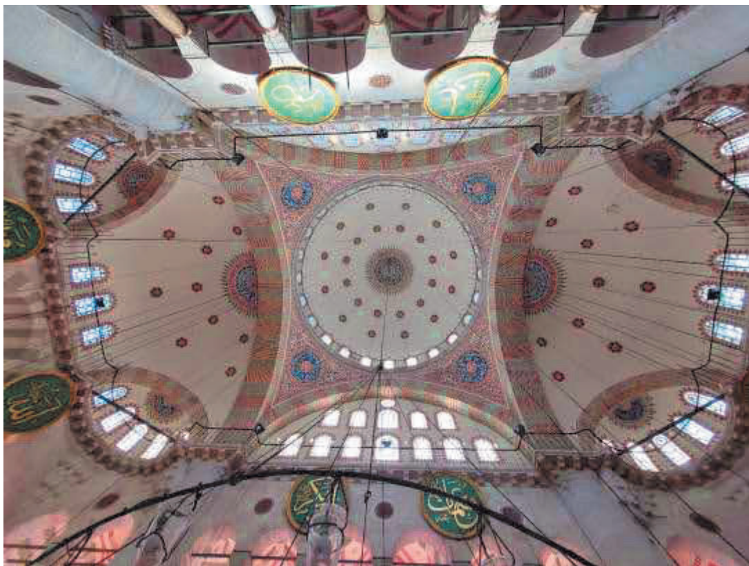
Fig. 8. Main dome with two semi-domes on the qibla direction axis
