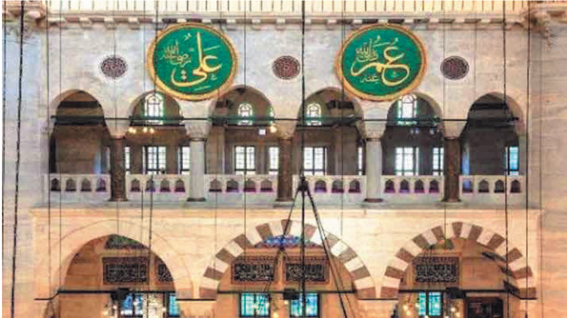
Fig. 9. Support walls and arch system on side facades (Tufan, 2021)
